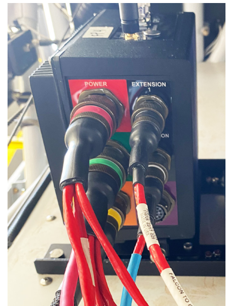
Foto 3-2: Install Image of Connections to Front of Falcon
